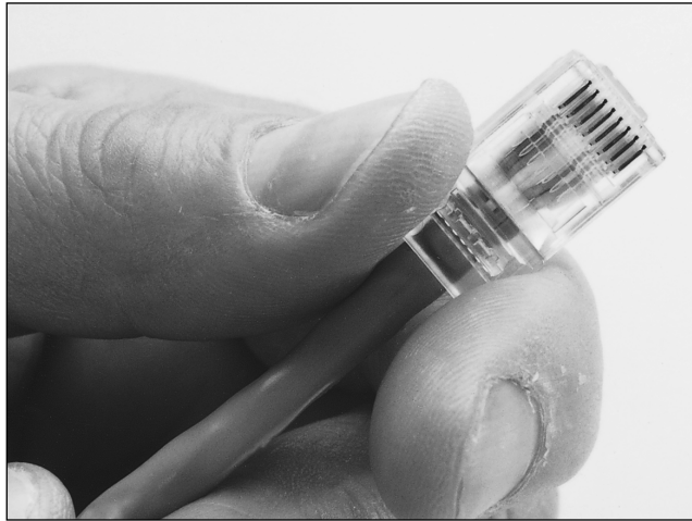
Figure 20.20 Push the RJ-45 connector into place, ensuring the cable pairs are ordered properly.
